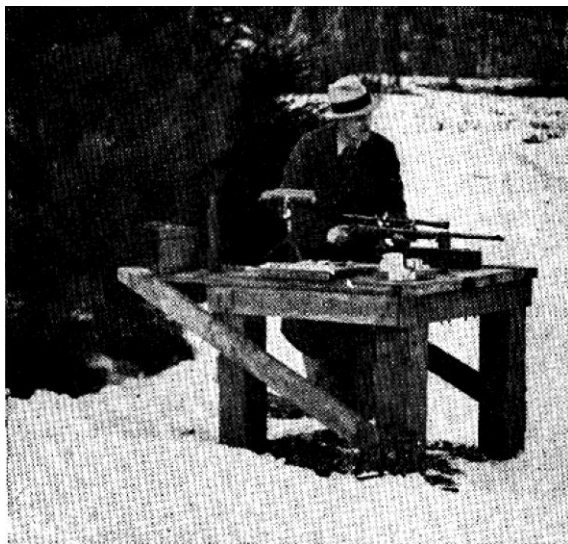
A good shooting bench is desirable for any form of test shooting. The above bench is made from 6 x 6-inch posts and set five feet into the ground, and not even a heavy Maine frost will throw it out of alignment. No nails are used in this bench—nothing but bolts and lagscrews
